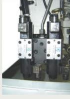
The hydraulic system employs Duplomatic (or equivalent) hydraulic solenoid valves for extremely smooth operation of the hydraulic system.
